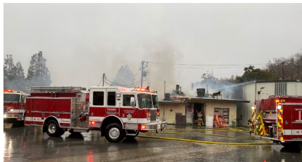
Willow Creek Wastewater Treatment Plant – Date of Loss 12-14-21
