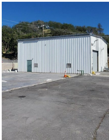
WCWWTP Demolition and Cleanup Complete
