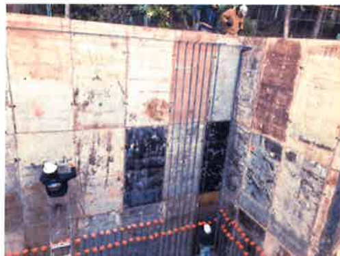
Outer form assembly near completion
