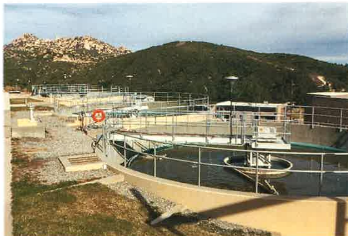
Grass Valley WWTP
