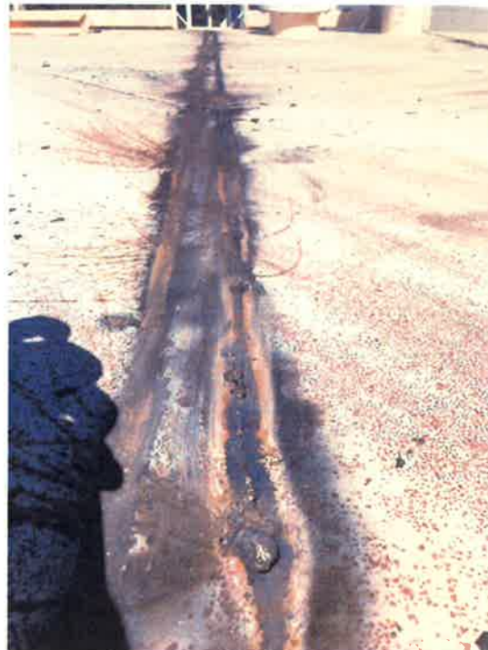
Welding view from the roof
