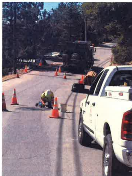
Manhole raising and traffic control
