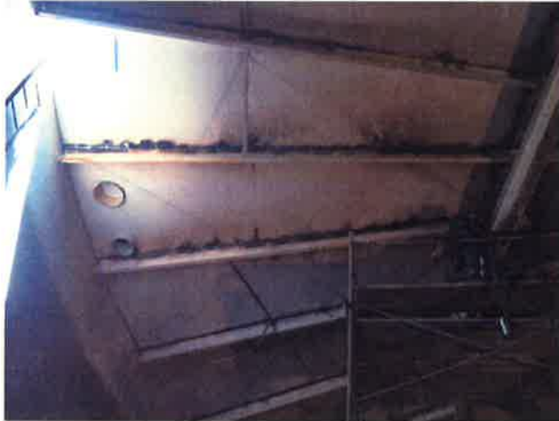
Welding view from the inside
