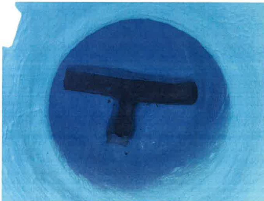
View of epoxy coating
